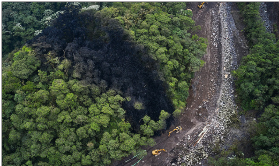
OCP Pipeline rupture, Ecuadorian Amazon, 2022. Photo: Mauricio Rosenfeld/Amazon Watch
