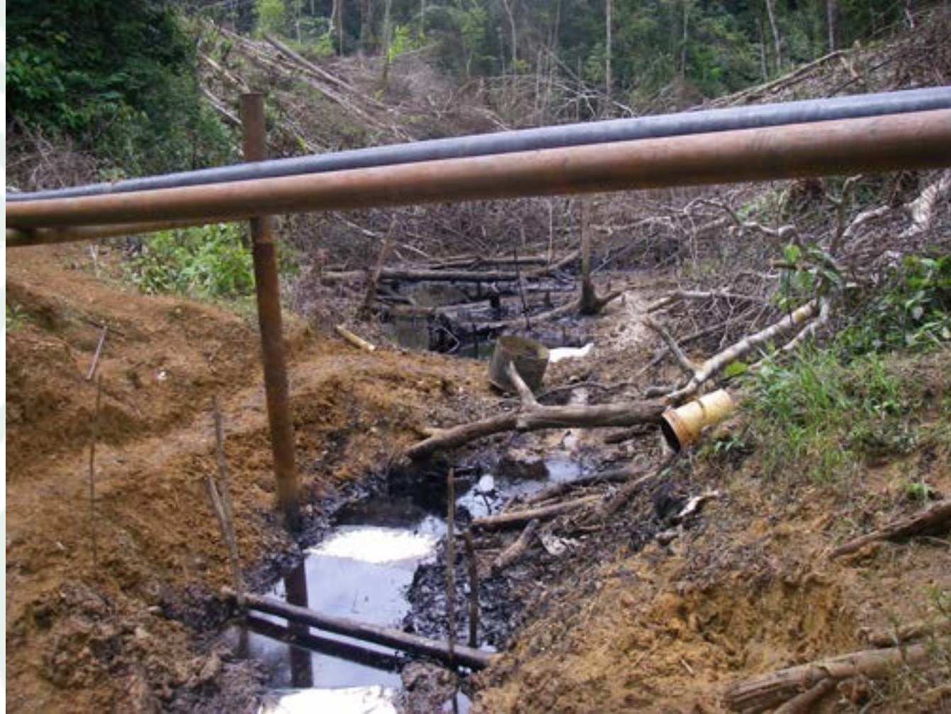
An oil spill on Timu Entsa creek in Oil Block 1-AB
