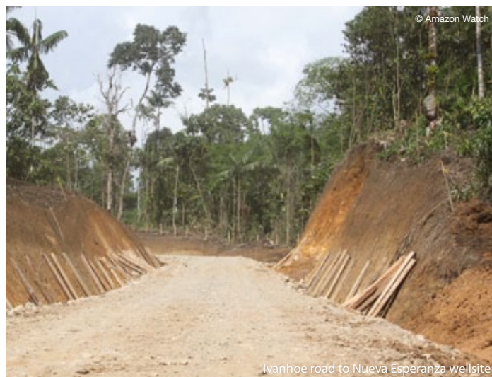
Ivanhoe road to Nueva Esperanza wellsite
